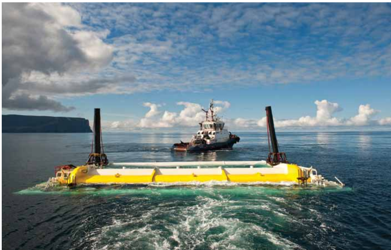
Oyster 800 wave energy device installation at European Marine Energy Centre in Orkney
