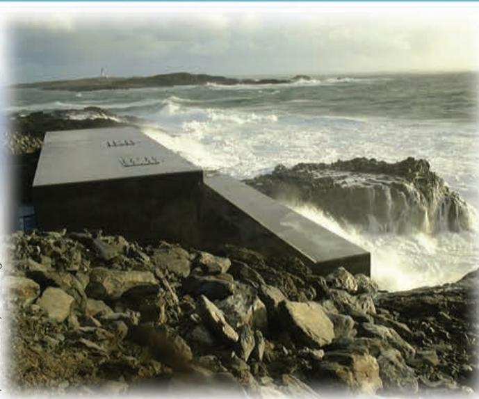
The LIMPET wave energy machine is on the island of Islay, off the west coast of Scotland. It started generating power for the islanders in 2000 and supplies power to about 350 homes. It was the World's first commercial wave energy machine.
