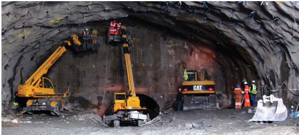
Glendoe's power cavern under construction
