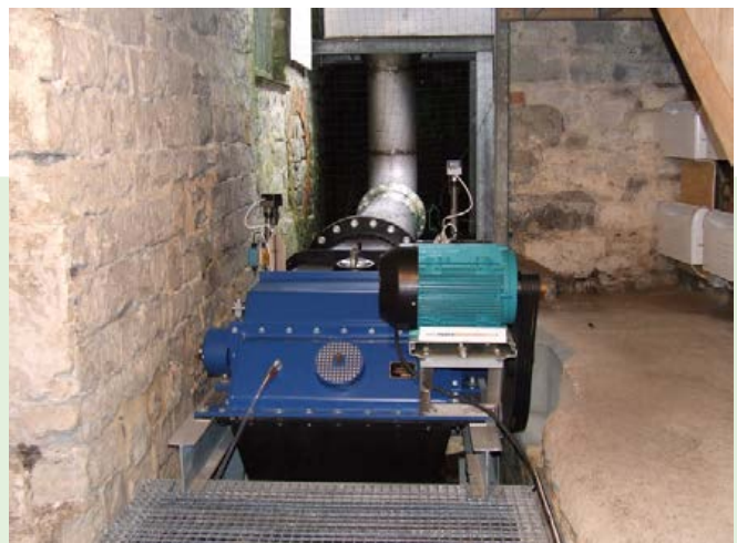
The installation and deployment of crossflow turbines at two former mill sites Images Courtesy of HydroGeneration Ltd
