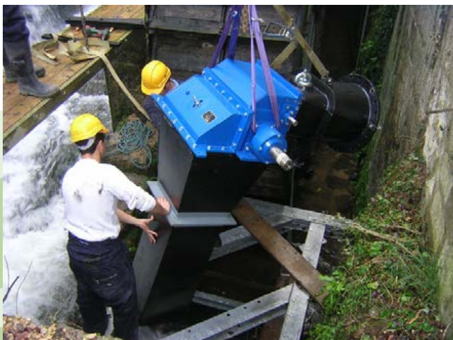
The installation and deployment of crossflow turbines at two former mill sites Images Courtesy of HydroGeneration Ltd
